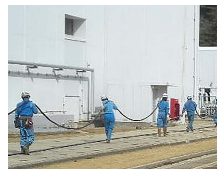
● Temporary power source cable installation at Fukushima Daini on March 13, 2011, two days after the disaster
