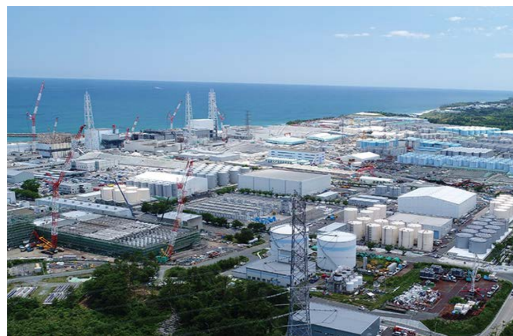
● Treated water storage tanks at Fukushima Daiichi Nuclear Power Station
