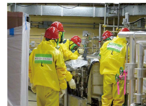
● Decontamination work for the decommissioning at Unit 1, Fukushima Daini on July 6, 2021
