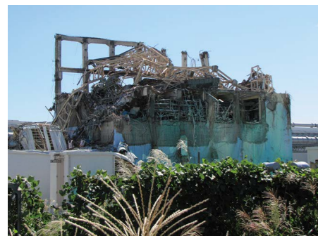
● Unit 3 Reactor Building at the time of the Fukushima Daiichi Nuclear Power Station Accident
