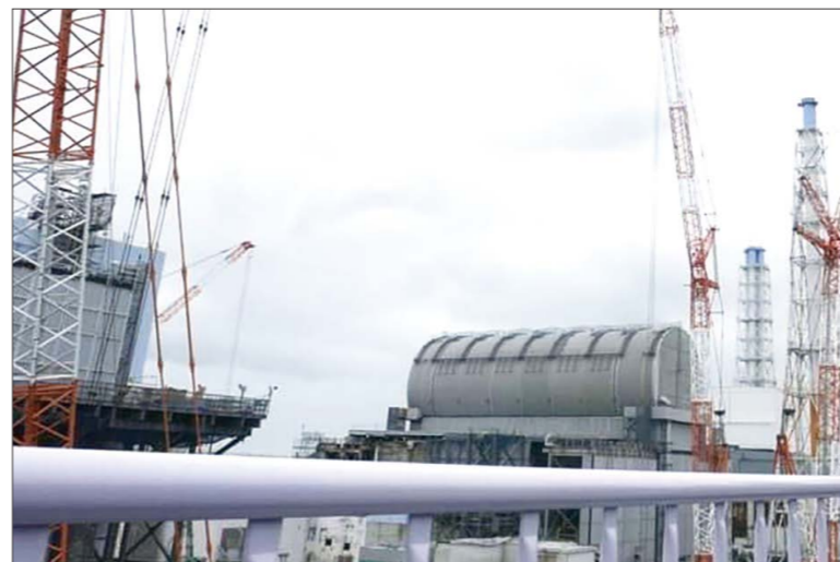
● A dome-shaped roof cover is installed on Unit 3, which caused the hydrogen explosion at the accident, to prevent the scattering of radioactive materials toward decommissioning. Many challenges continue
